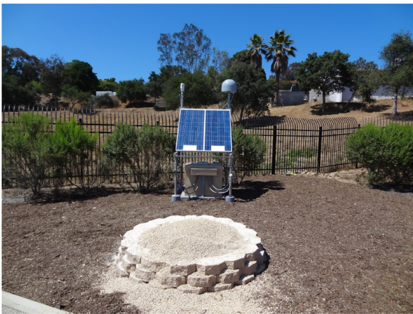
Figure 2. Station EOCG at the Santa Barbara Emergency Operations Center. Seismic vault is located in the foreground. Photo courtesy of Dan Determan, USGS. Photo was taken sometime between July and December 2014.
